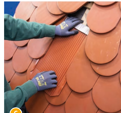
6 Check, if the opening of the support plate is hooked into the upper battening.
