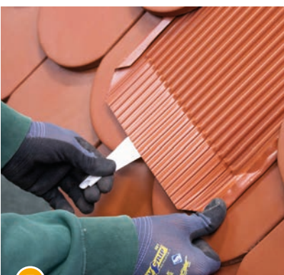
7 Completely peel off the cover of the adhesive tape from the back of the Beaver-Plate.
