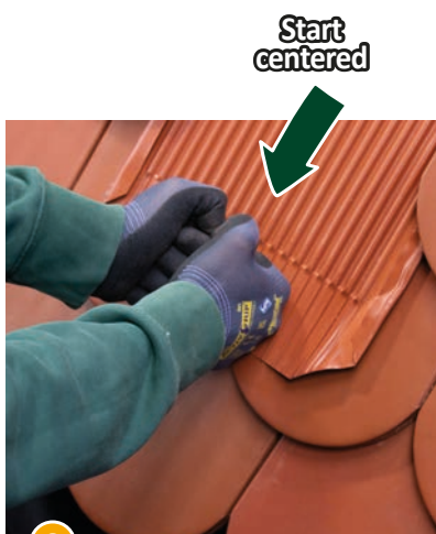
8 Starting from the center and working outwards, press down the Beaver-Plate firmly and ensure it is form-fitting.
