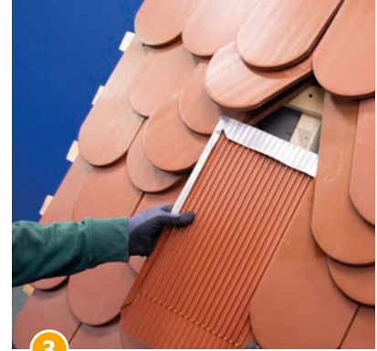
3 Align the opening of the support plate on the upper batten.
