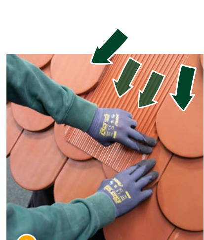
9 Make sure no water pockets can form in the upper and center part.
