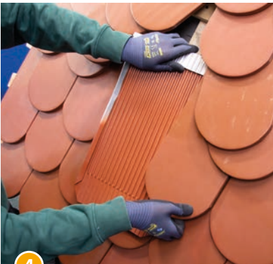
4 Lift the right tile and slide the Beaver-Plate underneath.
