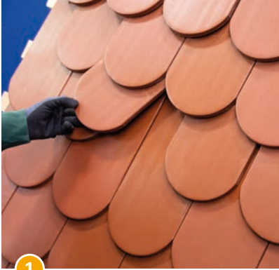
1 Remove the tiles in the installation area. Position the remaining tiles...
