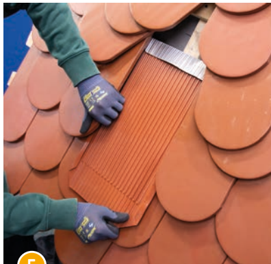
5 Lift the left tile and place it over the Beaver-Plate.
