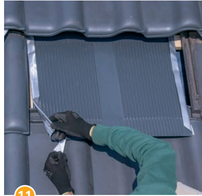
11 Completely peel off the cover of the adhesive tape from the back of the Beta-Plate.
