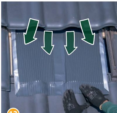
13 Make sure no water pockets can form in the upper and center part.
