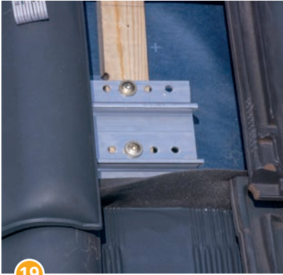
19 Fasten the base plate to the rafter with a minimum of 2 wood screws (at least 1 screw per horizontal row of holes) with a tightening torque of 10 Nm.
