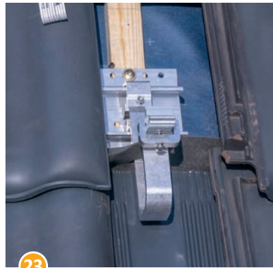
23 ...around the roof hook.
