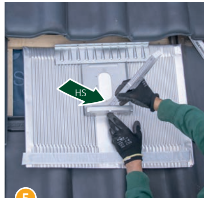
5 Height of tile (HT) = height of support plate (HS).
