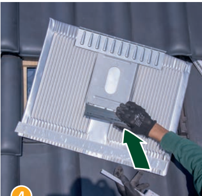
4 Adjust the height of the Beta-Plate by folding the support plate on the back.
