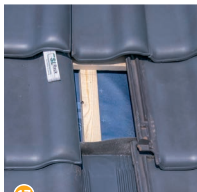
17 Remove the tiles above the Beta-Plate.
