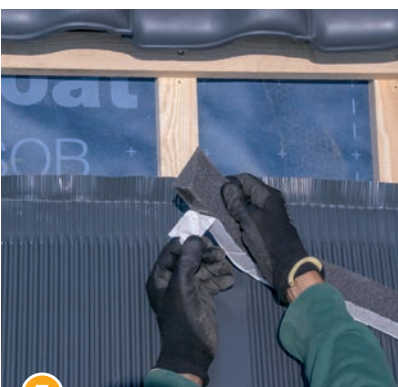
7 Peel off the cover of the adhesive tape from the back of the foam wedge.
