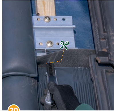
20 Cut the foam wedge at the position of the roof hook with an L-cut.
