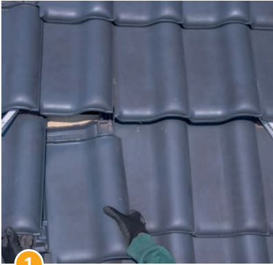
1 Remove the tiles in the installation area (max. 3 tiles). Position the remaining tiles...
