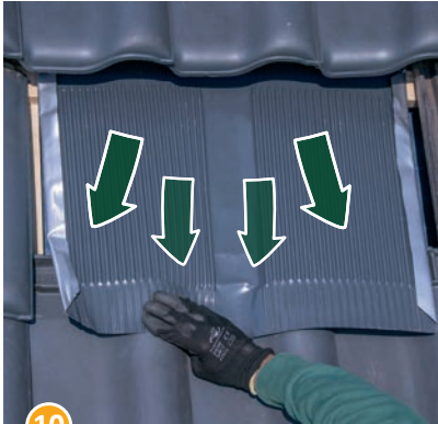
10 Press down on the bottom edge to roughly form-fit the Beta-Plate to the tiles.
