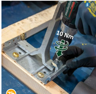
7b Fixate it by tightening the bolt with 10 Nm.
