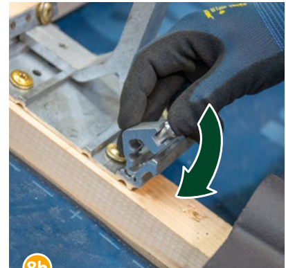
8b Optional: Hook the Potential Equalization Clamp into the bottom of the Alpha-Flex and tilt it forward.
