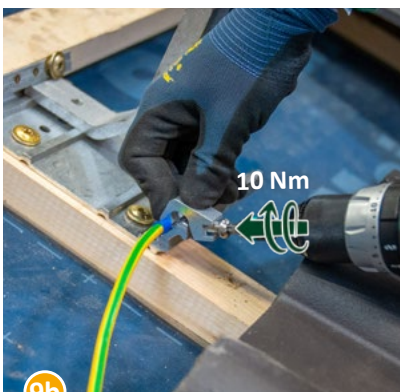
9b Insert the cable and fixate the position by tightening the bolt to 10 Nm.
