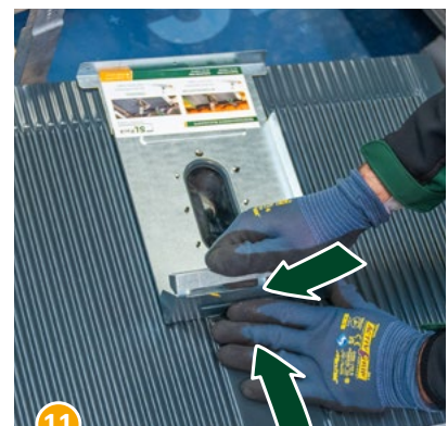
11 Adjust the height of the Alpha-Plate by bending the support plate on the back accordingly.
