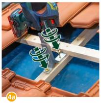
Attach the console with 2 wood screws. **Proceed to step 10.**
