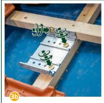
With the groove facing upwards, position Alpha-Flex on the roof batten, offsettig it left/right and attaching it with a min. of 3 wood screws.
