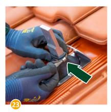
Additionally secure the top of the sealing sleeve by using the hose clamp (*Item no.* 11502-00-06). Place the clamp into the groove of the sleeve and tighten it.
