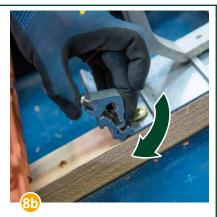
*Optional:* Hook the Potential Equalization Clamp into the bottom of the Alpha-Flex and tilt it forward.
