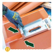
Adjust the height of the Alpha-Plate by bending the support plate on the back accordingly.
