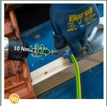
Insert the cable and fixate the position by tightening the bolt to 10 Nm.
