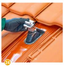
Slide the Clamp Combination over the console, drop the rail on top and push it in. Adjust the height through positioning the Clamp Combination on the console.
