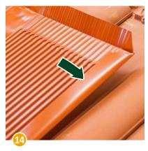
Align the Alpha-Plate and ensure that there are no unintentional indentations in the top and center area, which could lead to the formation of water pockets.
