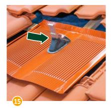
Place the opening in the support plate on the upper horizontal batten and put the Alpha-Plate with its riveted sealing sleeve over the console.
