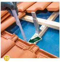
Determine the height of the roof tile (DH), that needs to be compensated.
