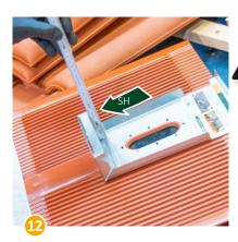
Height of roof tile (DH) = Height of support plate (SH).
