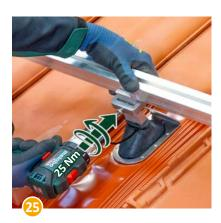
Now fixate the positon by tightening the bolt to 25 Nm.
