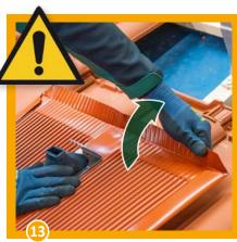
Press the rear sheet metal edging slightly backwards, to ensure full coverage of the upper upstand.
