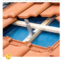
Slide the long side of the console against the roof batten, which serves as a reference point.
