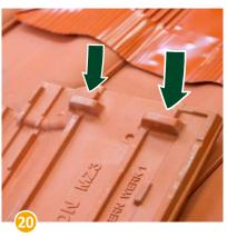
The locking lugs on the back of the clay tiles that need to be reinstalled, ...
