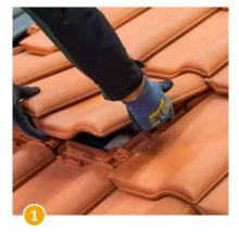
Remove tiles in the installation area (max. 3 tiles) and position the remaining tiles
