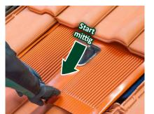
Starting from the center and working outwards, press down the Alpha-Plate firmly and form-fitting ...
