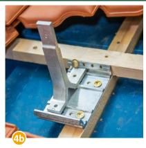
Insert the long side of the console into the upper groove of the Alpha-Flex.
