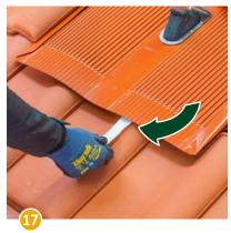
Completely peel off the protective paper from the adhesive strip on the back of the Alpha-Plate
