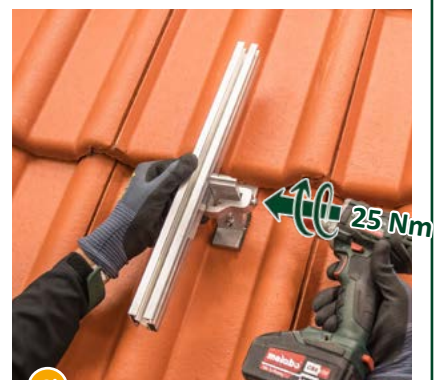
12b Fixate the Clamp Combination by tightening the bolt (25 Nm) – done!
