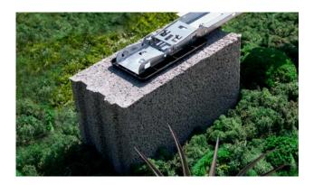
1. Place the hollow core blocks in the position of the Fast Flat Base Plates, according to the information from the design software.
